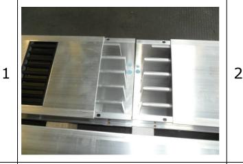
Insert the monoblock joint with the screw's head on the PE side.
