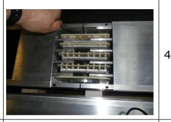
Insert the PE joint with steel springs facing towards the interior of the duct.
